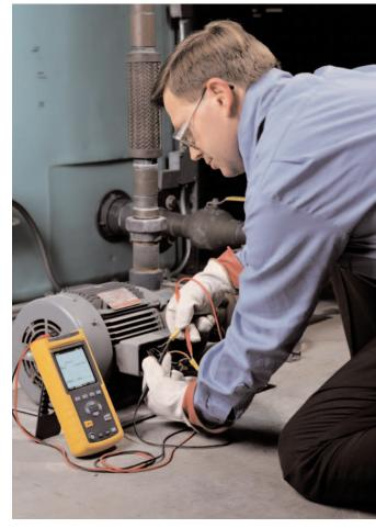
should also be checked. This can be done with direct voltage measurements or with infrared thermometers. Readings that are much higher than the ambient temperature, or that are higher than other phases, can indicate loose or otherwise bad connections.
