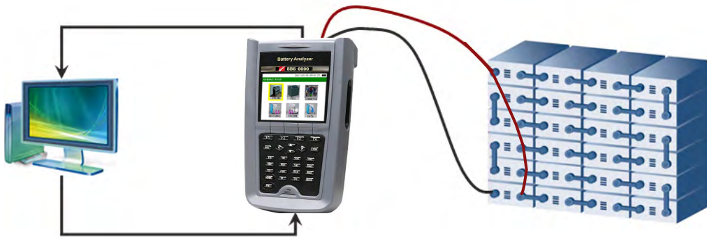
Battery resistance testing
