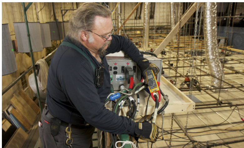
On a set for television production at CBS Studios, Roger Lattin checks the current on an overhead power supply with his Fluke 376 Clamp Meter.
