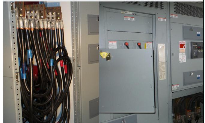
Incoming line connection and main breaker cabinets were also fitted with 24-inch windows
