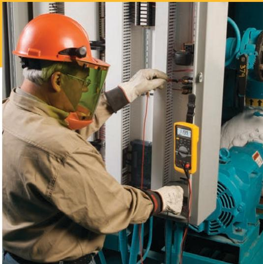
Always wear approved personal protective equipment (PPE), including arc rated clothing, leather over rubber gloves, safety glasses, and an arc-rated face shield or hood, both with hard hat and hearing protection.
