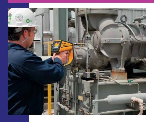
Specifically, plant operations and maintenance personnel can maximize the reliability of production assets using predictive maintenance (PdM) techniques that monitor the condition of production assets while they operate. The goal is to detect impending failures of assets and correct those developing problems in order to avoid unplanned shutdowns.
