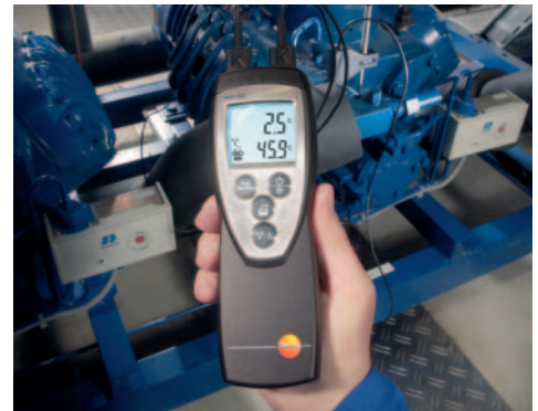
Simultaneous measurement of superheat and subcooling in refrigeration plants
